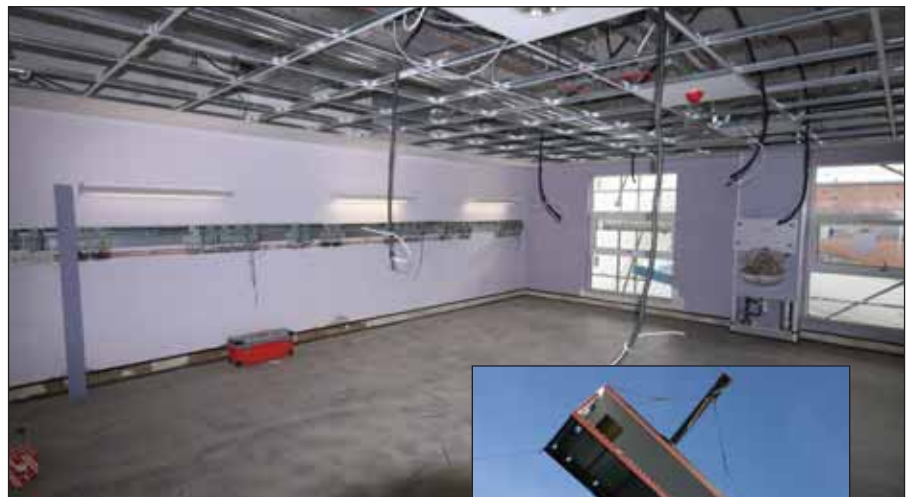
Once the modules were in place, MTX's team began installing the remainder of the internal mechanical and electrical services.
