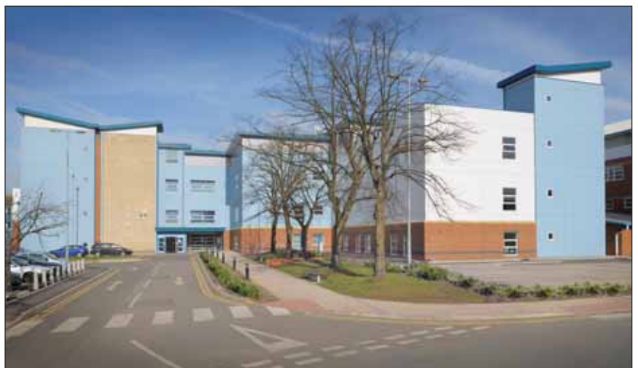
The new modular building was completed to a tight schedule.
