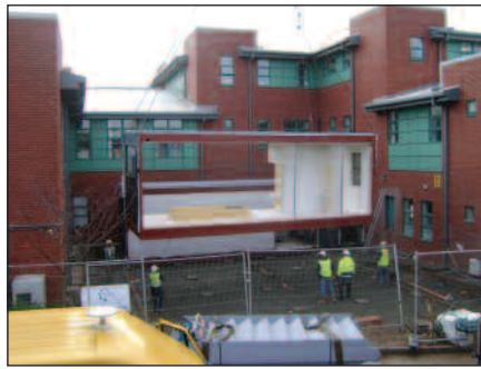
Some of the key project stages: the groundworks completed; a module being lifted into position and, with all 15 modules in place, the building begins to take proper shape.
