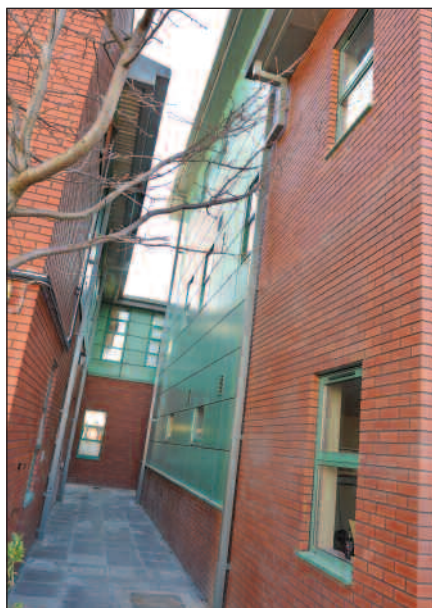
The new building had to be constructed within a tight three-sided courtyard location with some elements within two metres of existing walls.
