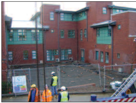
Some of the key project stages: the groundworks completed; a module being lifted into position and, with all 15 modules in place, the building begins to take proper shape.
